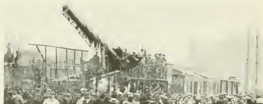
280 M/M GUN WHICH BOM- BARDED AMIENS. CAPTURED BY AUSTRALIANS. RANGE: 30 MILES
